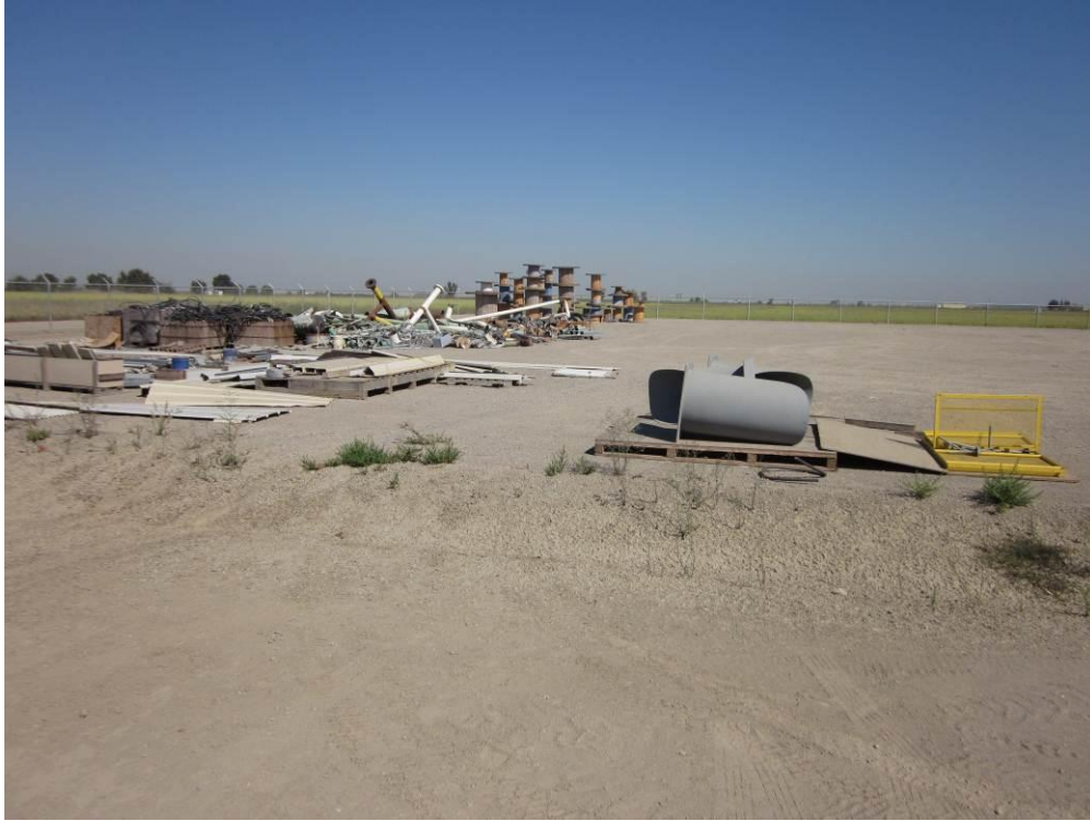
Photo 4: Construction-related materials remain in the northern portion of the Compressor Station site.
